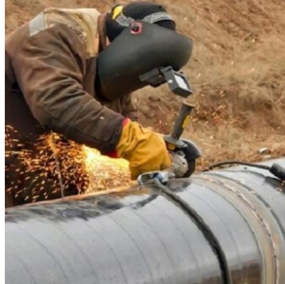
Piping design & Installation
